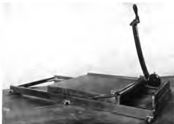
Fig. 1. Finger Guard for Paper Cutter. (General Electric Co.)
